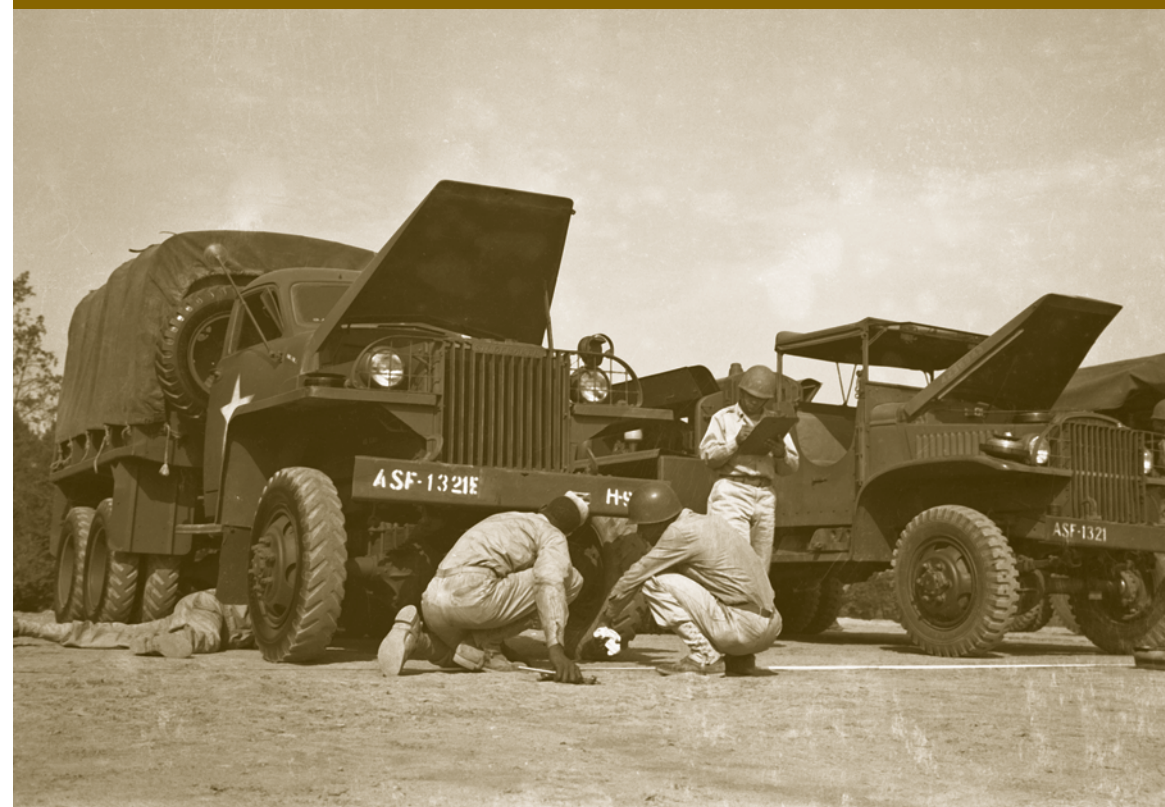
Engineers of the 1321st during a vehicle inspection.
