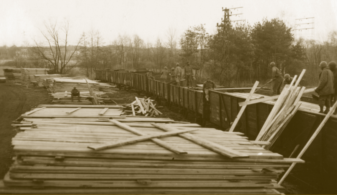
Soldiers unloading timber at the lumber yard in Vincey, France, 9 February 1945.
